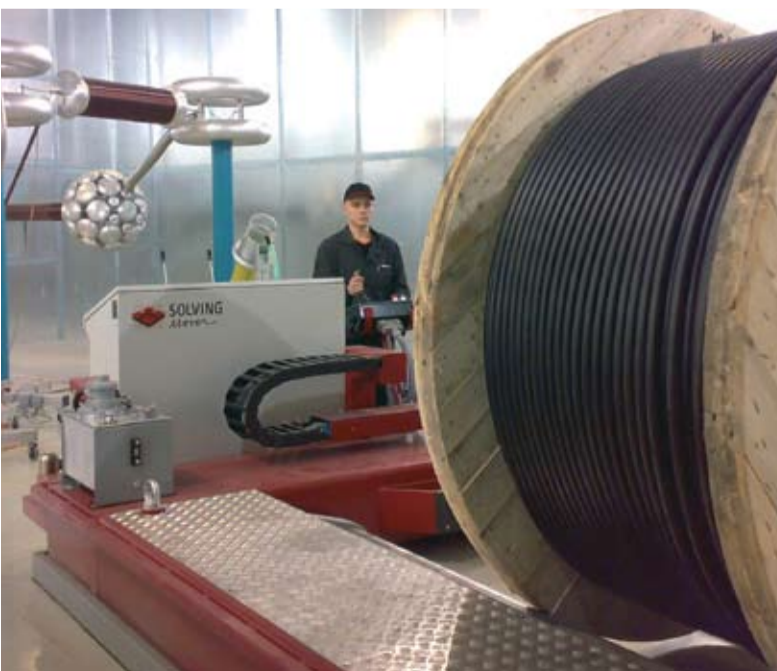
Using a Solving air film Mover cable drums are moved safely in a high voltage test laboratory.
